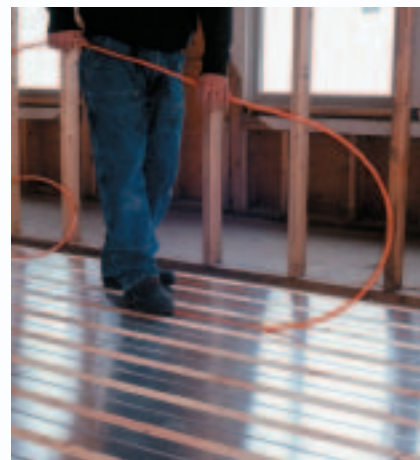
RAUPANEL is a great option for retrofit and new construction applications because it is installed without the concrete overpour.
